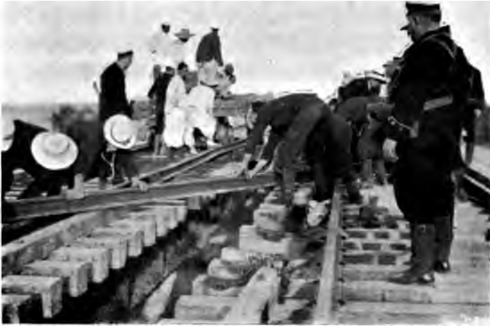
REPAIRING THE LINE.
